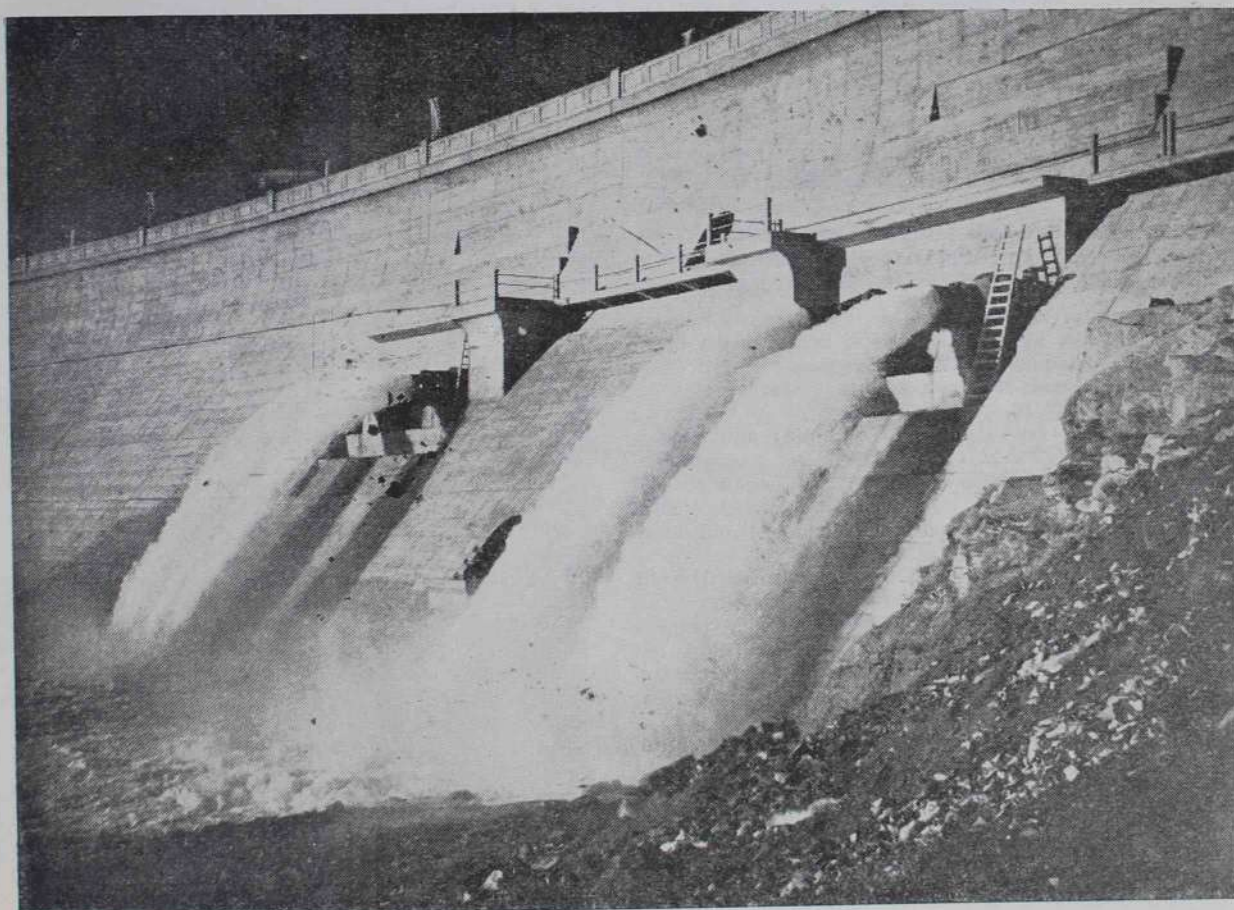
View of the "El Nihuil" dam, located in the province of Mendoza, 75 kms. south of San Raphael, storing the waters of the Atuel River. This dam, recently inaugurated, is one of the most important ever built in Argentina. It contains a reservoir constituted by a lake with a surface of 7.500 hectares, and a water storing capacity of 260.000.000 cubic meters. Its maximum height is of 26 meters
