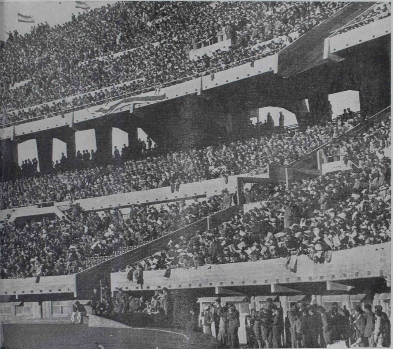
View of a section of the imposing stadium belonging to the foot-ball club River Plate. This monumental structure, has a sitting capacity of over 90.000 spectators and will accommodate about 120.000, when a new section now in construction is added to it. In the River Plate stadium, resembling an enormous horseshoe, are usually held most of the international foot-ball matches, played in the Argentine Capital
