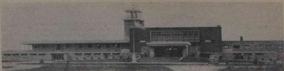
A partial view of a block of the principal building of the City of Córdoba airdrome, which counts with some of the most up-to-date appliances
